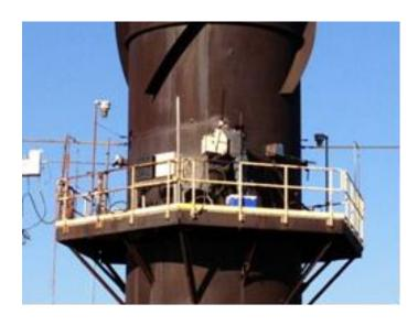
Monorail literally held in place with baling wire...supporting the weight of a sample train box over 100 feet above ground.
