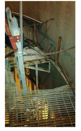
OSHA regulations for a ladderway floor opening or platform opening: "Every ladderway floor opening or platform shall be guarded by a standard railing with standard toeboard on all exposed sides (except at entrance to opening), with the passage through the railing either provided with a swinging gate or so offset that a person cannot walk directly into the opening."
